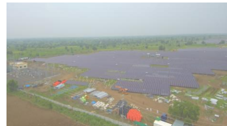
Solar panel – Open Access Agreement
