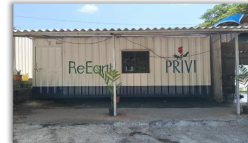
Mahad Highway Police Helpline Center
